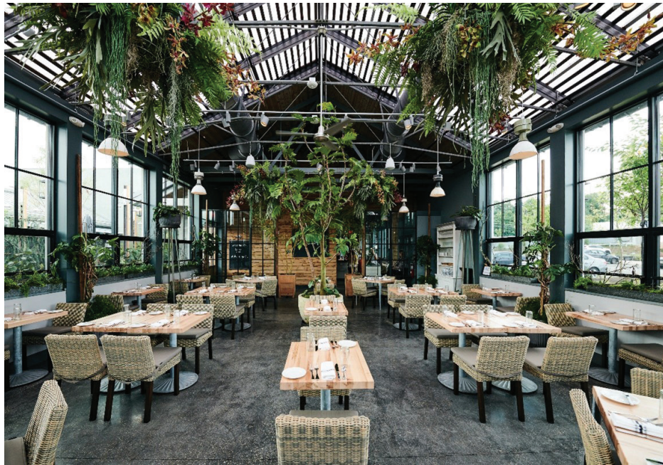
Terrain Gardens at Devon Yards in Devon, Pennsylvania, reused steel trusses from a University of Maryland structure built with bolted connections for easy disassembly and then reconnected them in the new space to form the framework of their new venue. (Photo credit: David Greer.)
